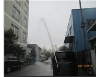
Photo of fire safety equipment Testing fire hydrant.JPG
